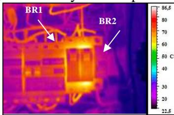
Fig.4: Termogram of breakers in electric switchgear
