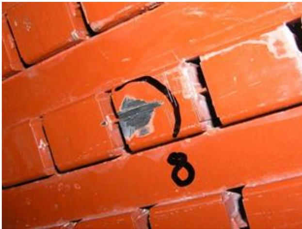
Fig. 5. Defect made by a grinding machine.
