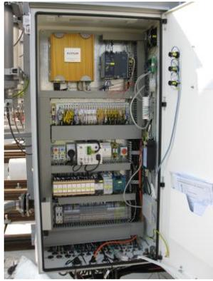
Fig. 1. Example of the the MS 3000 installed at CEPS transformer
