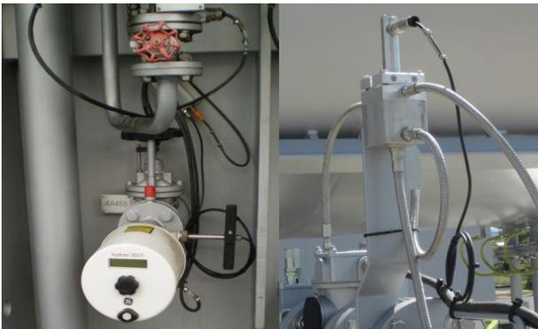
Fig. 4. Moisture and gas sensors (left) and Buchholz gas sensor (right)
